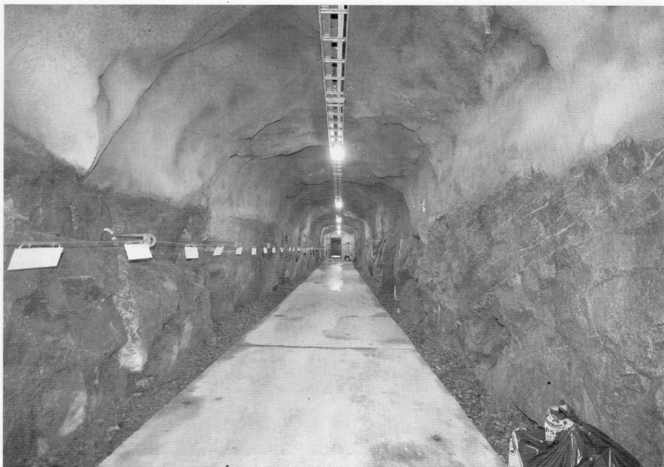
Entrance Tunnel to the Civil Defence Bunker at Enköping - Photo By Dan McKenzie.
